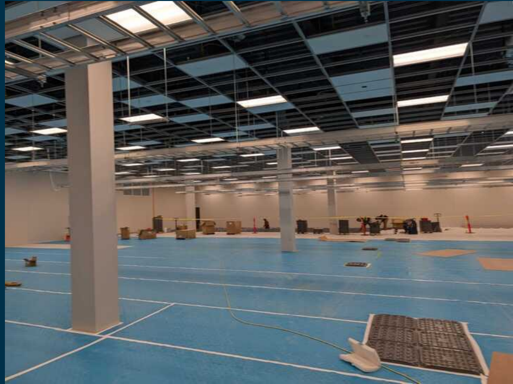
October 2025 Raised floor install
